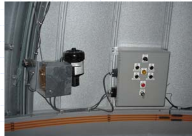
Right: Shutter/Drop-out Control Box up-graded with RF receiver for remote operation.
