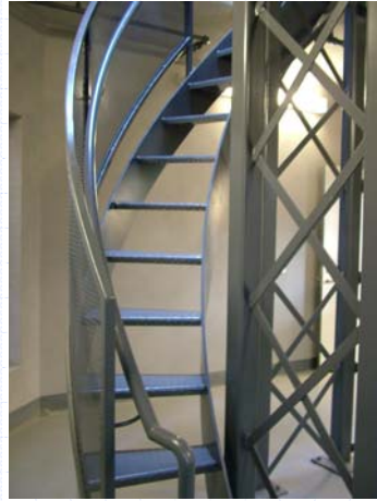
New stairway installed December 2006.
